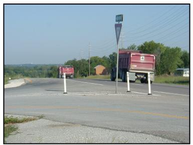
FIGURE 76. MoDOT MAL with median channelization
