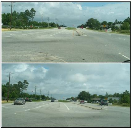
FIGURE 101. Parallel offset left-turn lanes at US-421 & Golden Road (northbound view)
