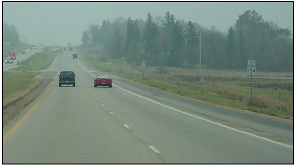
FIGURE 104. Conventional advance intersection guide signing along US-52 (94)
