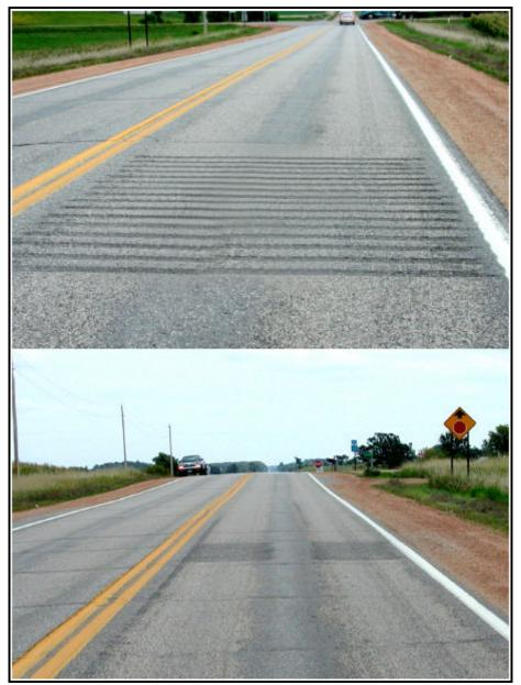
FIGURE 30. In-lane intersection approach rumble strips (47)
