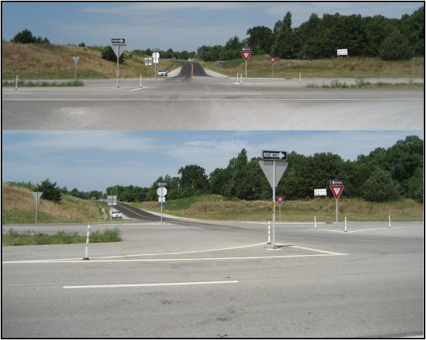
FIGURE 29. Photos of MoDOT Type II median opening with median channelization
