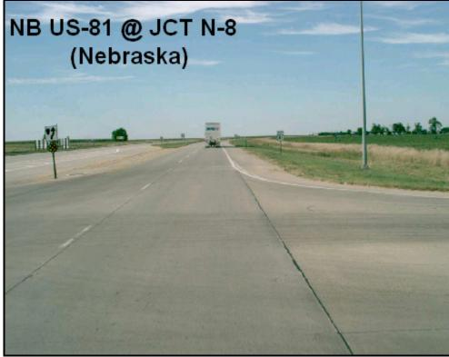
FIGURE 98. Opposing through driver's perspective of offset left with surfaced median
