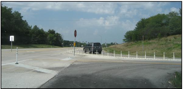
FIGURE 20. Right-turn acceleration lane delineators used in Missouri
