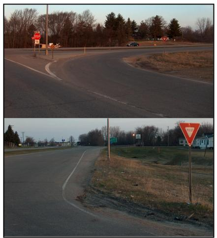
FIGURE 17. Right-turn acceleration lane in Minnesota
