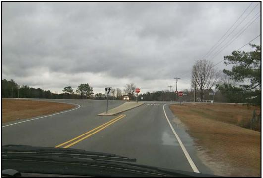
FIGURE 31. Splitter island on minor road approach to an expressway intersection (50)
