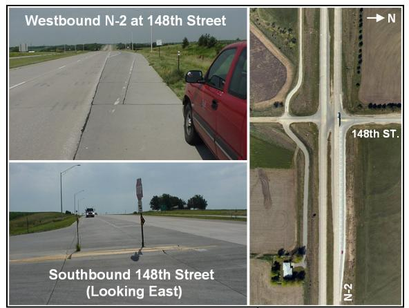
FIGURE 86. Offset right-turn lane at N-2 & 148<sup>th</sup> Street – near Lincoln, NE
